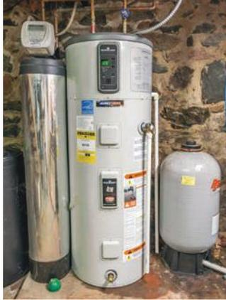
**Double duty.** Hybrid electric heat pump water heaters use the surrounding warm air to heat water. They also offer premium features such as a user-friendly display, vacation mode, and Internet of Things (IoT) capabilities that allow unit monitoring and control from anywhere.
