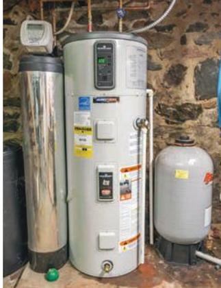
**Double duty.** Hybrid electric heat pump water heaters use the surrounding warm air to heat water. They also offer premium features such as a user-friendly display, vacation mode, and Internet of Things (IoT) capabilities that allow unit monitoring and control from anywhere.
